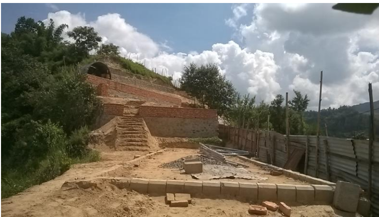
Satya Uddham land being readied for construction
